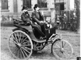
In 1886, Karl Benz produced his first car, the Motorwagen with a steering tiller in the middle. Early cars like the 1896 Ford Quadricycle and the 1901 Oldsmobile Curved Dash used the center-mounted tiller.
